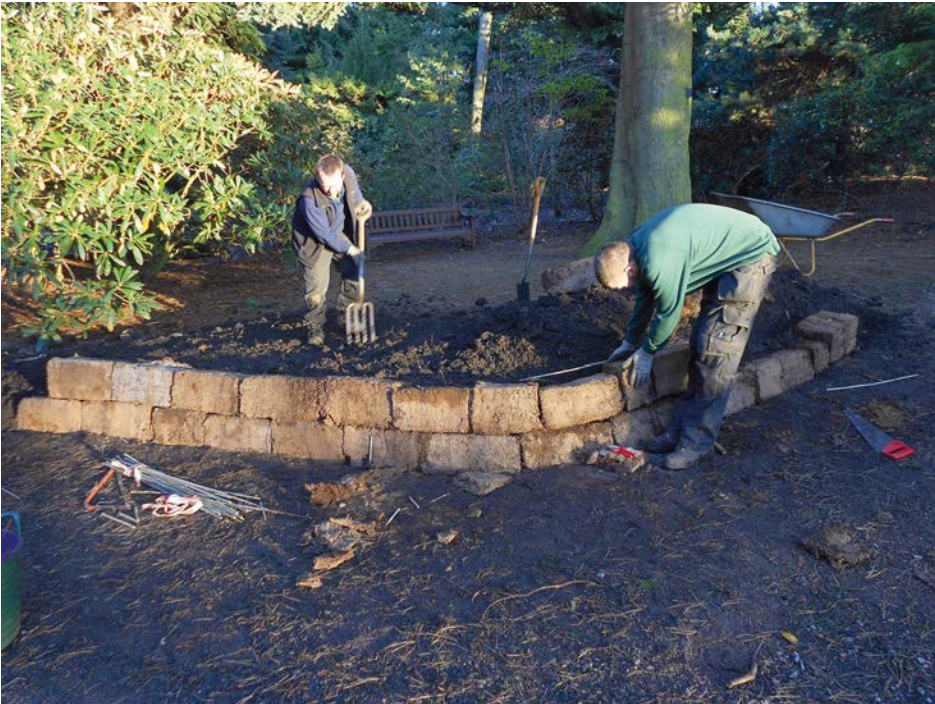
Fig. 9 Peat Wall construction. Photo: David Knott.
