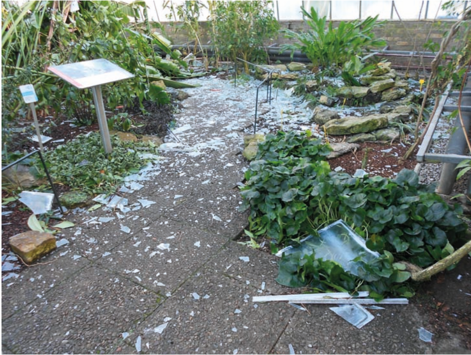
Fig. 4 Glass fragments in the Lowland Tropics glasshouse at RBGE caused by the storm on 3 January 2012. Photo: David Knott.
