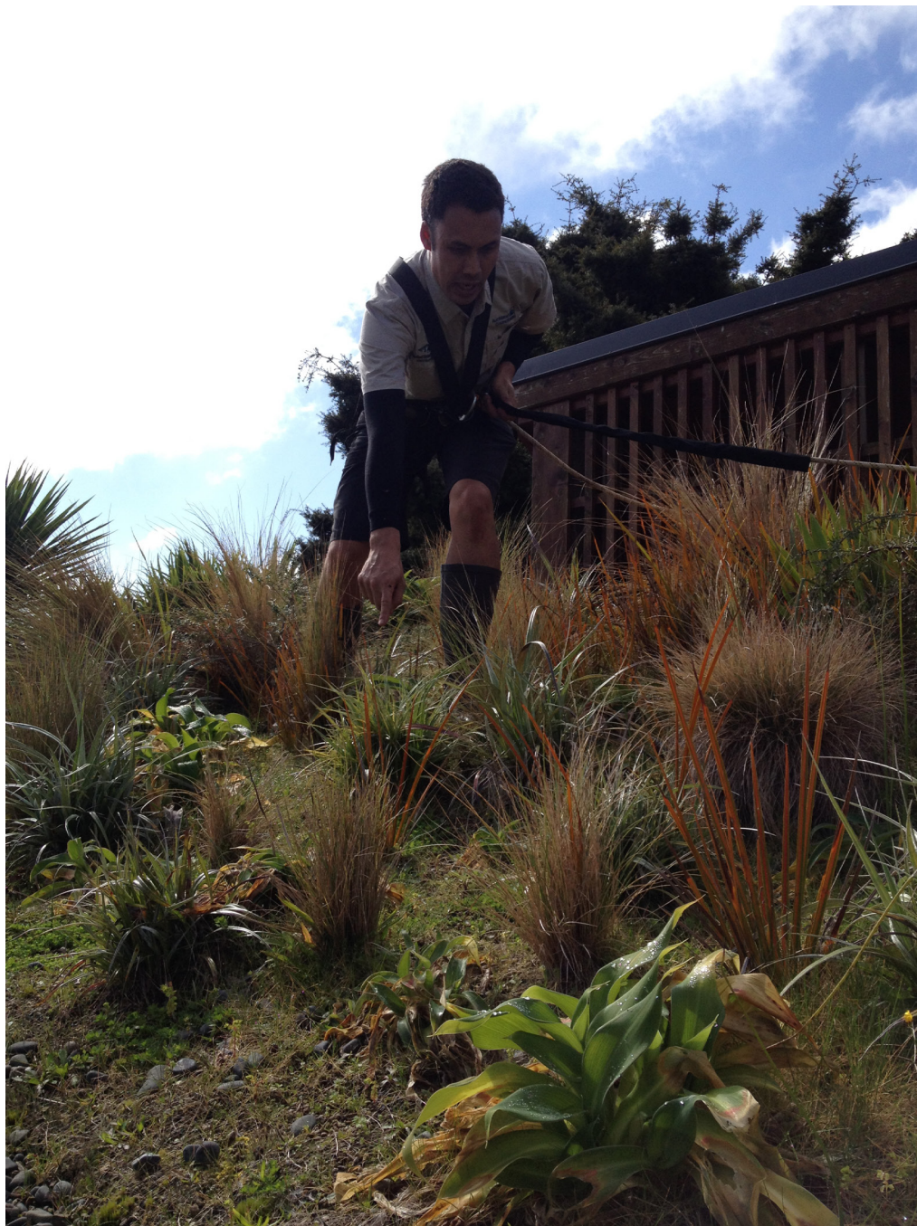
Fig. 3 Staff maintaining the roofs through weeding, removing spent flowers and fertilising. Photo: Emma Bodley.
