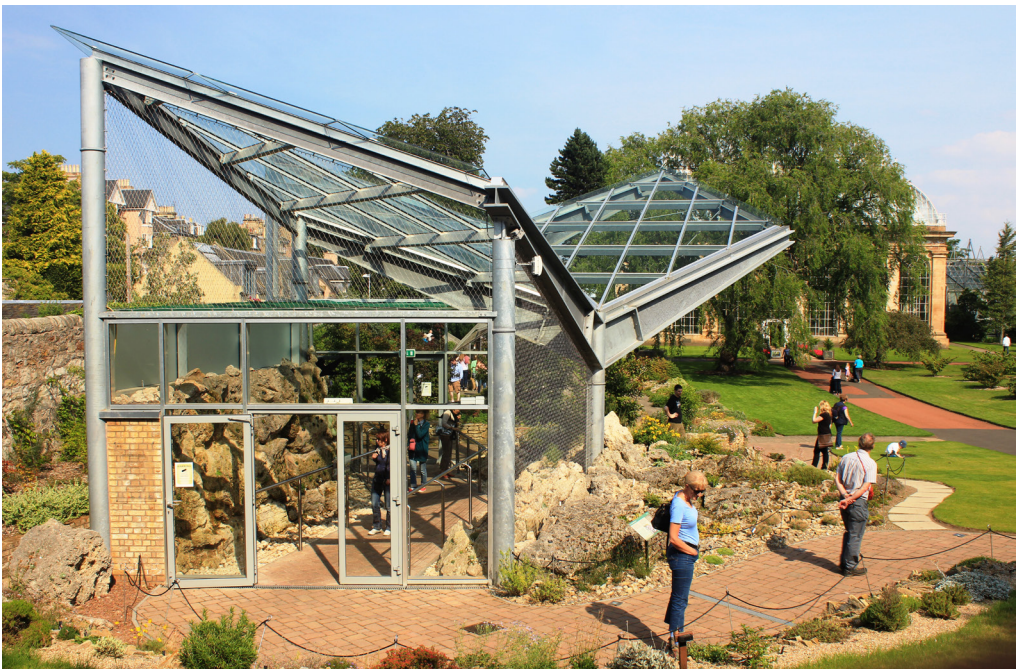
Fig. 11 The new Alpine House has a clear but solid roof and is open on all sides to allow ventilation while protecting plants from rainfall. Photo: David Knott.
