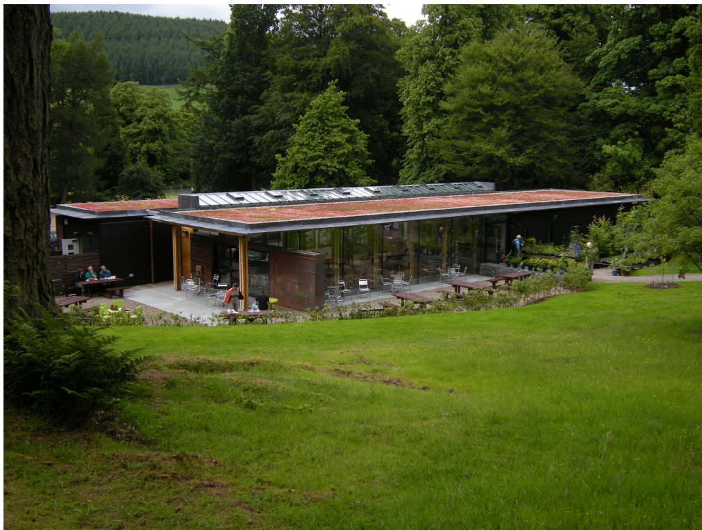
Fig. 15 The Visitor Centre at Dawyck with its sedum roof. Photo: David Knott.
