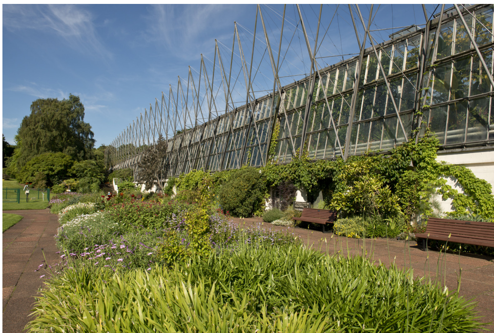
Fig. 3 The Front Range was completed in 1967 and is Grade A listed. Photo: Lynsey Wilson.
