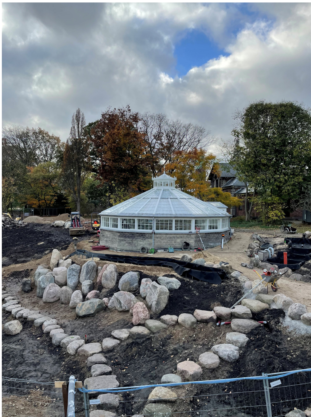
Fig. 1 The construction site of the new Rhododendron Quarter. Photo: Tina Jørgensen.
