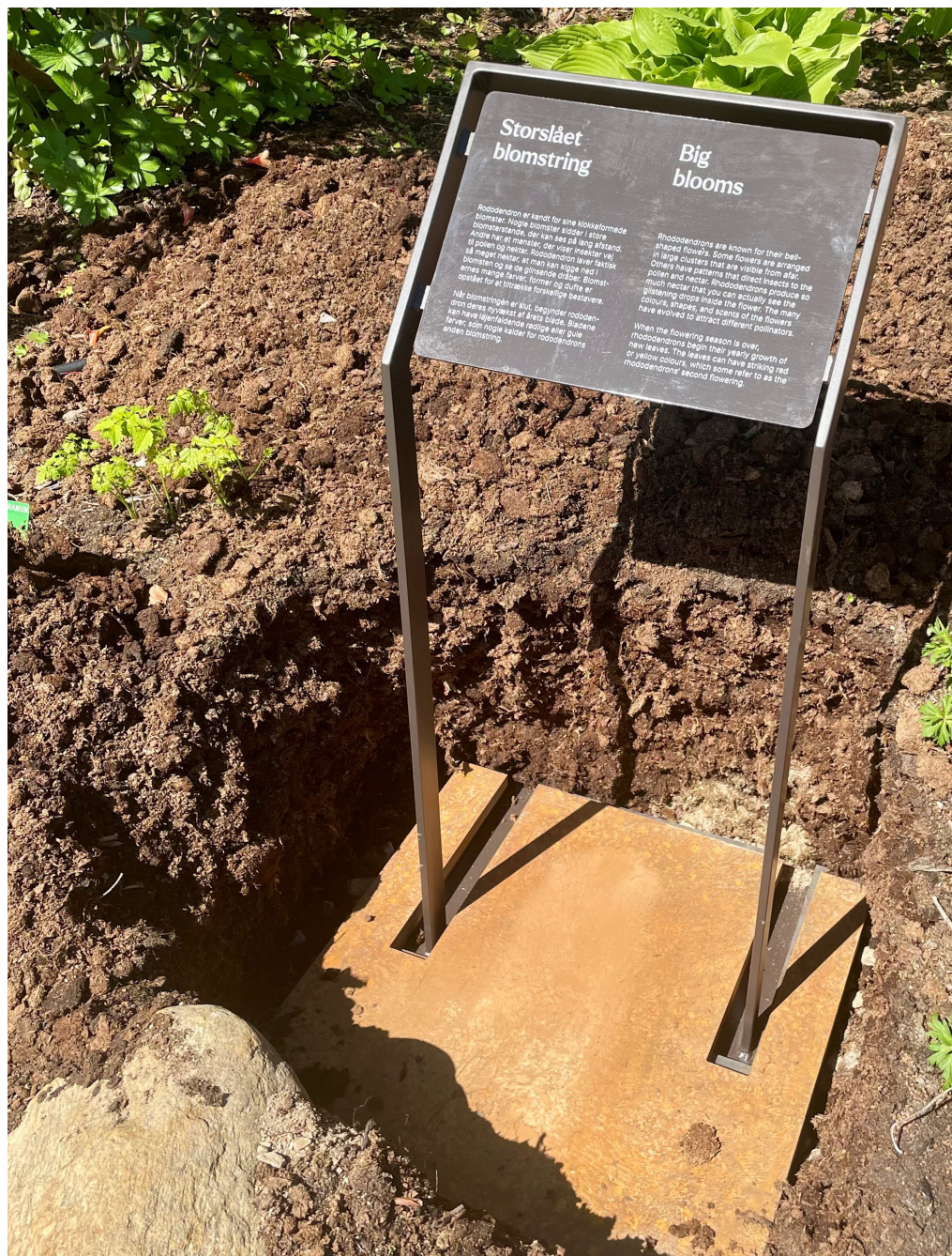
Fig. 7 Construction of the panels and their metal frames. The heavy base ensures they are stable but also portable when necessary. Photo: Tina Jørgensen.
