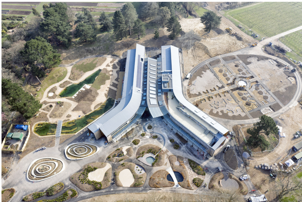
Fig. 5 RHS Wisley's Hilltop Building – The Home of Gardening Science is surrounded by three new gardens. The Wellbeing Garden is to the front, the Wildlife Garden on the left and the World Food Garden on the right. Photo: RHS/ Chris Gorman.
