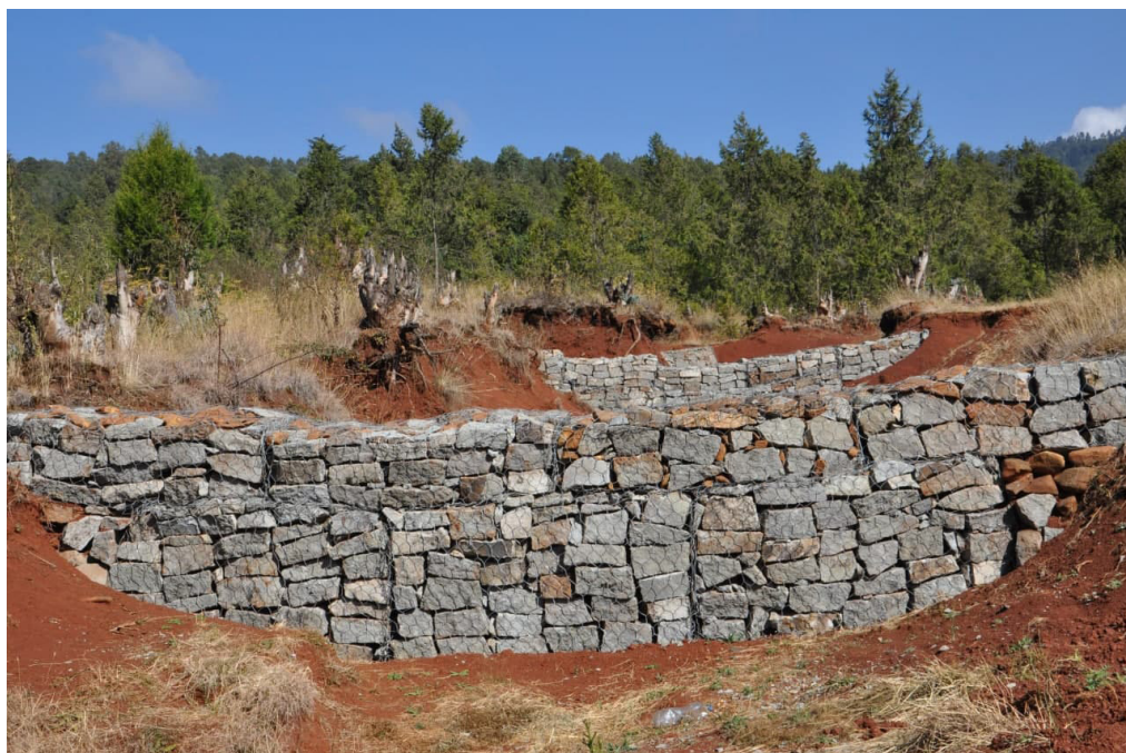
Fig. 8 Gabion check dam (strong enough to resist the force of runoff). Photo: Communication unit, GBG.
