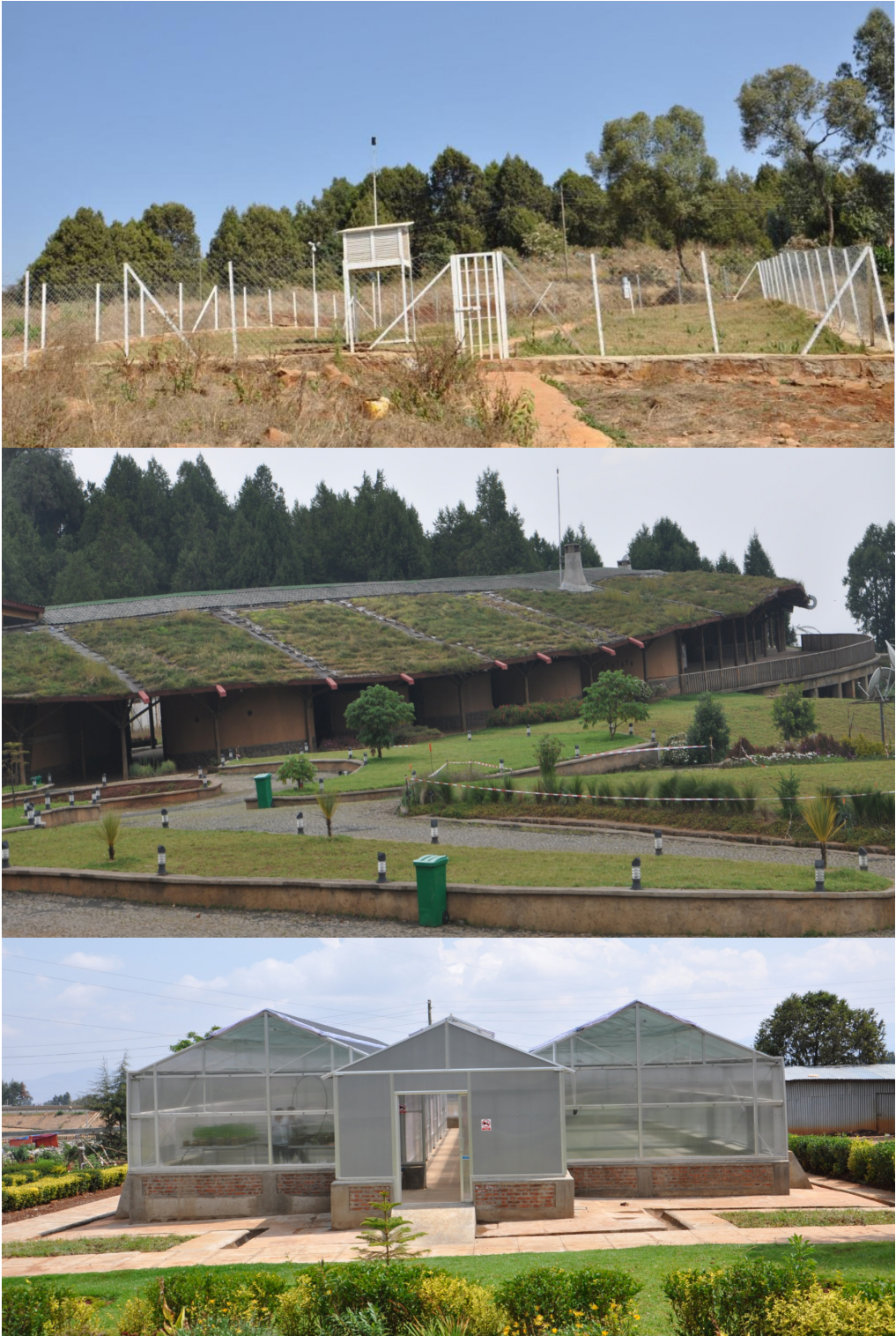
Fig. 2 Examples of new infrastructure: (top) weather station (centre) research facility buildings (bottom) greenhouse. Photos: Communication unit, GBG.
