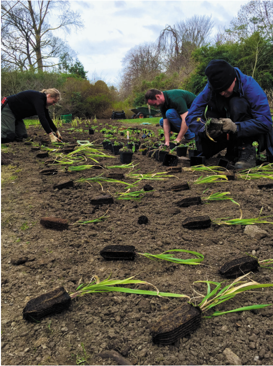
Fig. 14 Members of the horticulture team lay out the young plants before planting into the amended soil of the raingarden. Photo: David Kelly, Heriot-Watt University.
