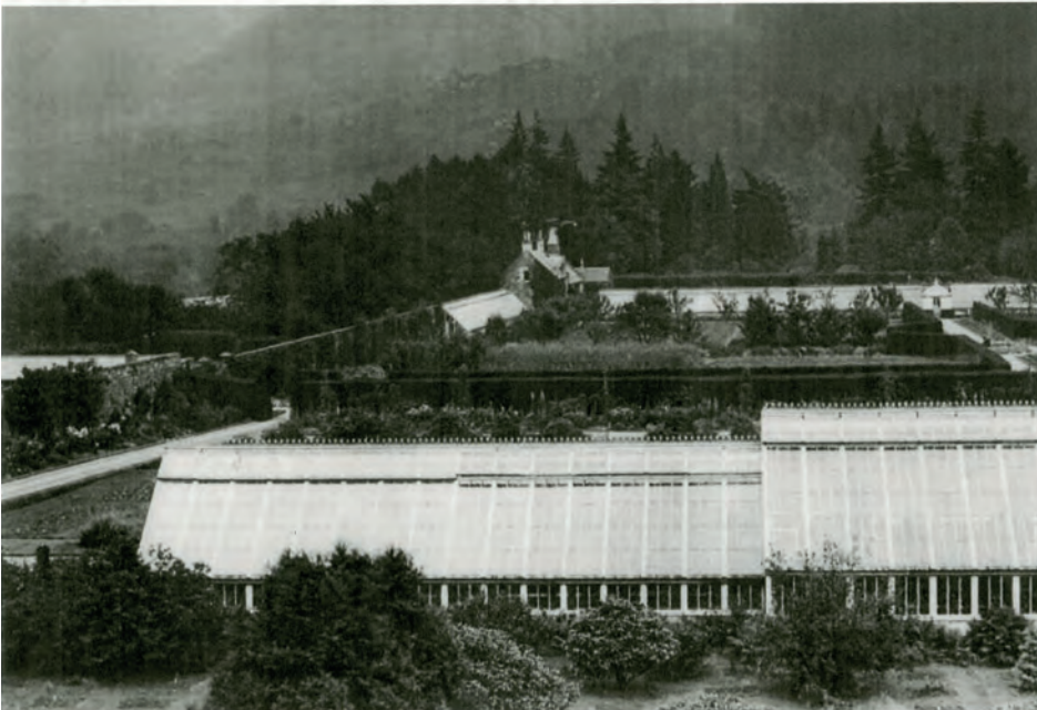
Fig. 4 Black-and-white view from west (fragment, undated). Miscellaneous photograph in Benmore Curator's office, kindly made available by Peter Baxter. It is quite conceivable that this image may post-date the demolition of the winter garden.
