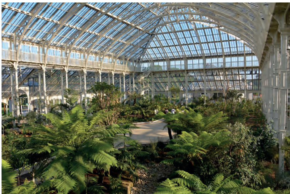
Fig. 1 The centre section of the Temperate House shortly after reopening in May 2018. Photo: R. Hilgenhof.
