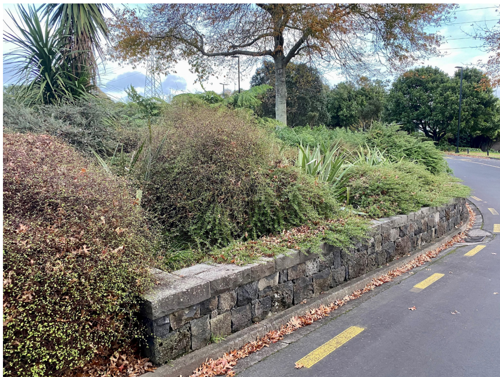
Fig. 11 The now well-established rain garden in 2023 in the main car park at ABG. Photo: Emma Simpkins.
