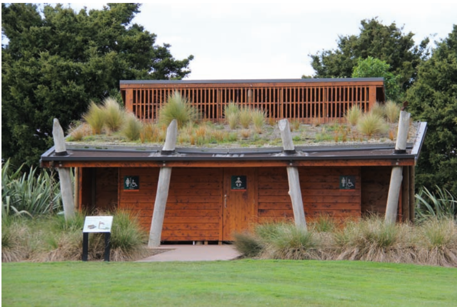
Fig. 15 Austrostipa stipoides and other native plants on the green roof at ABG. Photo: Jack Hobbs.
