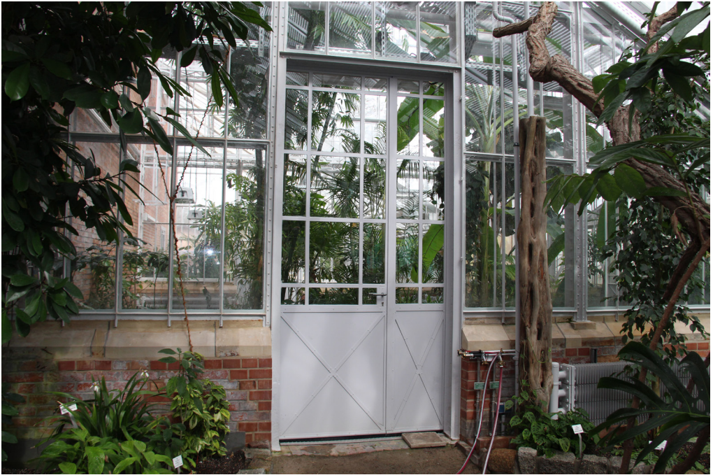
Fig. 16 View from the tropical house towards the palm house after renovation, with planting not yet complete: (right) trunk which would be used to display epiphytes; (bottom right) the old radiators. Photo: P. König.
