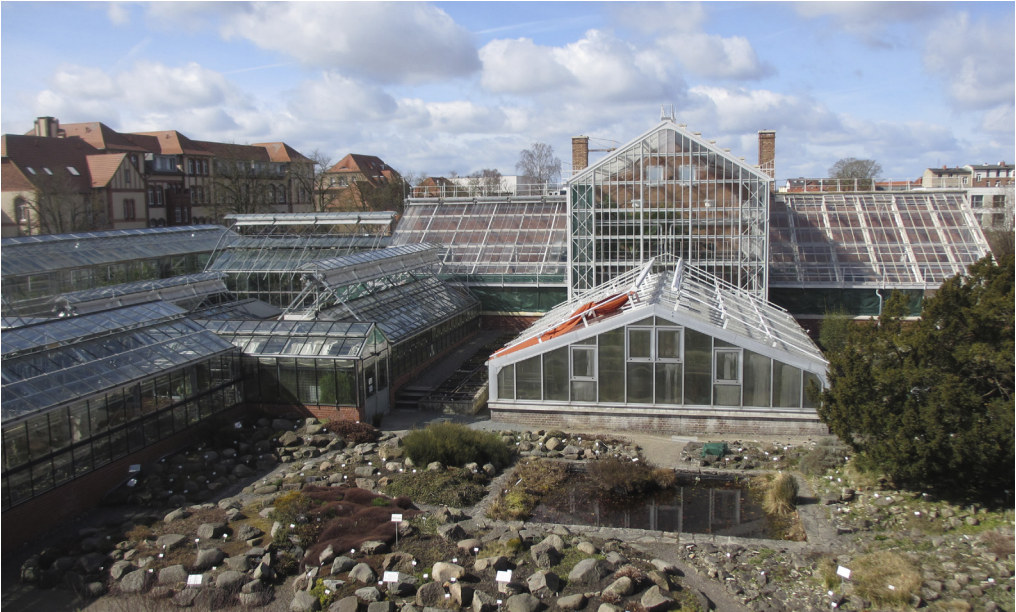
Fig. 18 A 2022 view of the greenhouse complex with the renewed historical section (two rebuilt chimneys). The aquatic plant house (erected in 1960, overhauled in 1997) is in the foreground, with the show house, succulent house and other greenhouses (1950s to 1962, demolished and rebuilt in 2010–2012) on the left. Photo: P. König.
