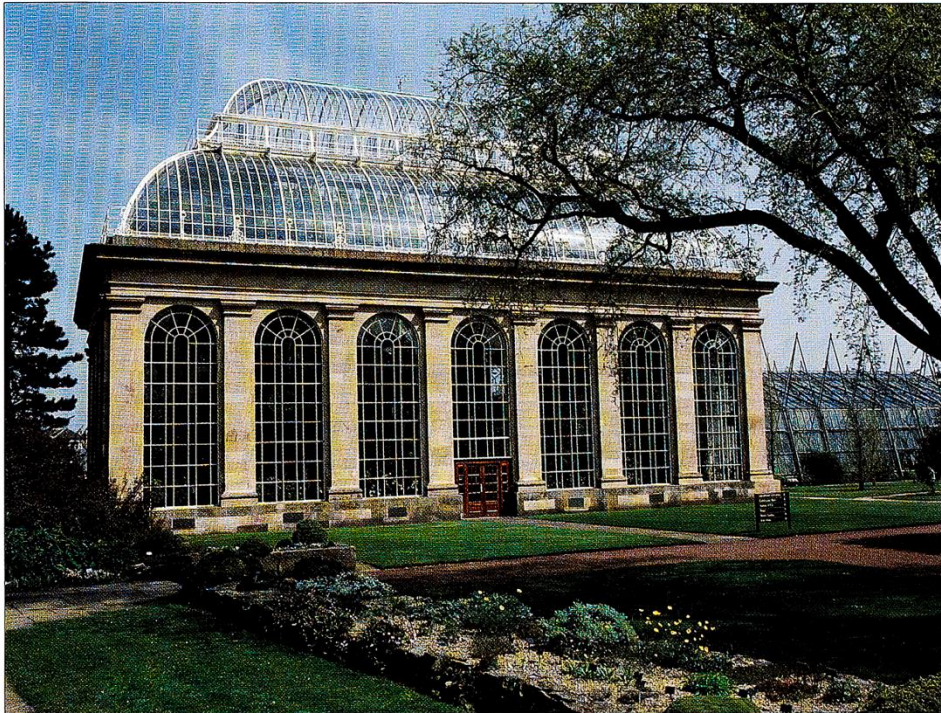
Plate 5a. The exterior of the Temperate Palm House, Royal Botanic Garden Edinburgh.
