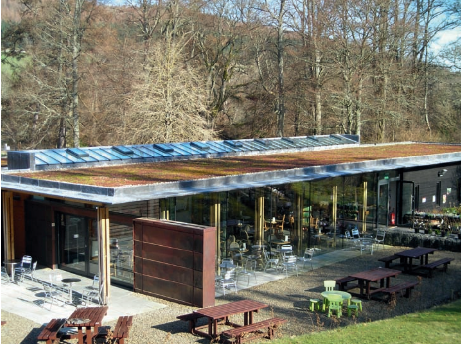
Fig. 4 The sedum roof attracts wildlife and insulates the building while absorbing rain run-off. Photo: Graham Stewart.
