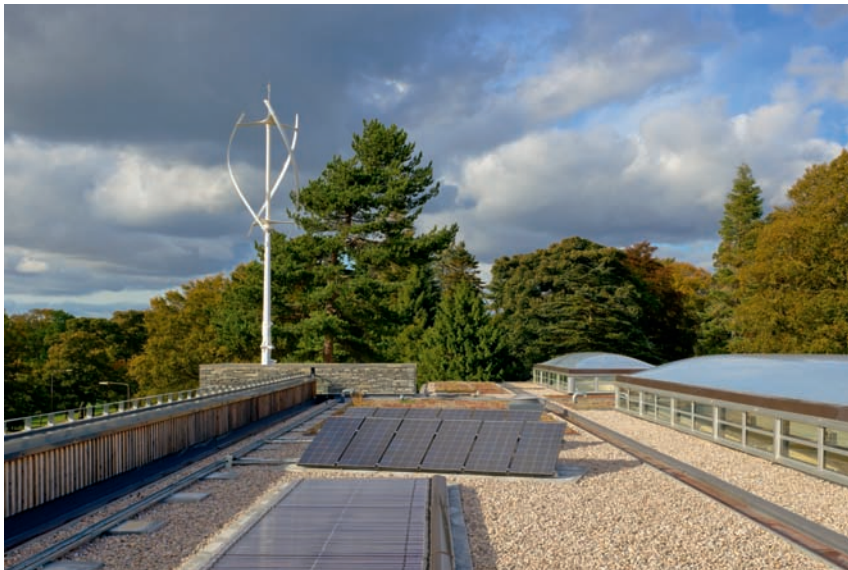
Fig. 6 Solar panels and heat exchangers installed on the roof of the John Hope Gateway Visitor Centre. The sedum roof and EFTE 'pillows' can also be seen. Photo: Matt Laver, architectural photographer.
