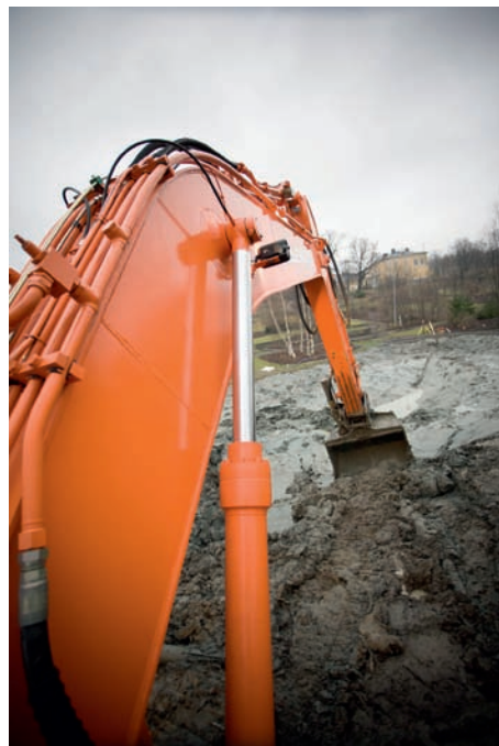
Fig. 14b Dredging the pond in January 2008. The work was scheduled for mid-winter with the expectation that the frozen ground would support the heavy machinery but the winter of 2007–2008 was one of the mildest ever recorded and the soil never froze properly. See Fig. 3 for the rebuilt pond. Photo: Mikko Paartola.
